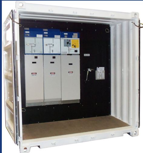
33000V 400A ring main unit mounted in 10ft sea container
